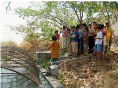
Greywater collection for irrigation
